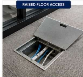
RAISED FLOOR ACCESS Take a clear photo of any raised floor boxes or access points.
